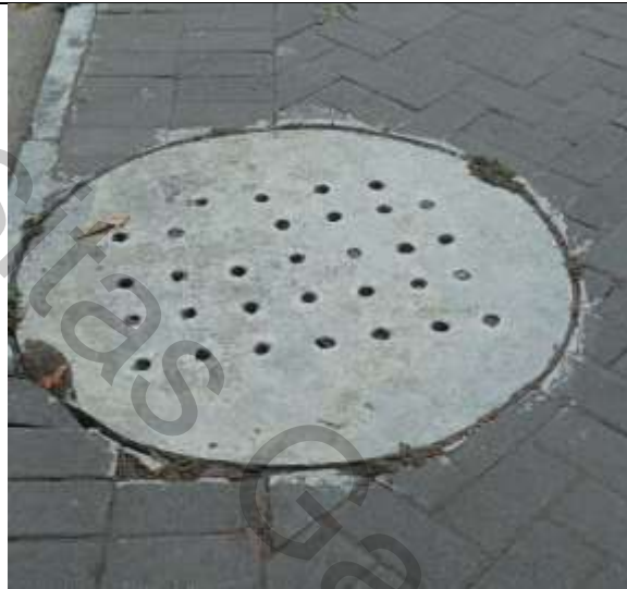
15(a) Infiltration Well in Faculty of Cultural Science
