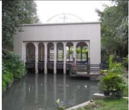
15(s) Stormwater retention in Pascasarjana School
