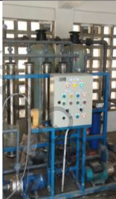
Figure 11 Greywater Installation (with Panel Control) in Faculty of Engineering
