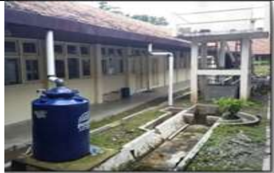
15(m) Injected Rain Water Harvesting in Department of Civil Engineering and Environmental Engineering
