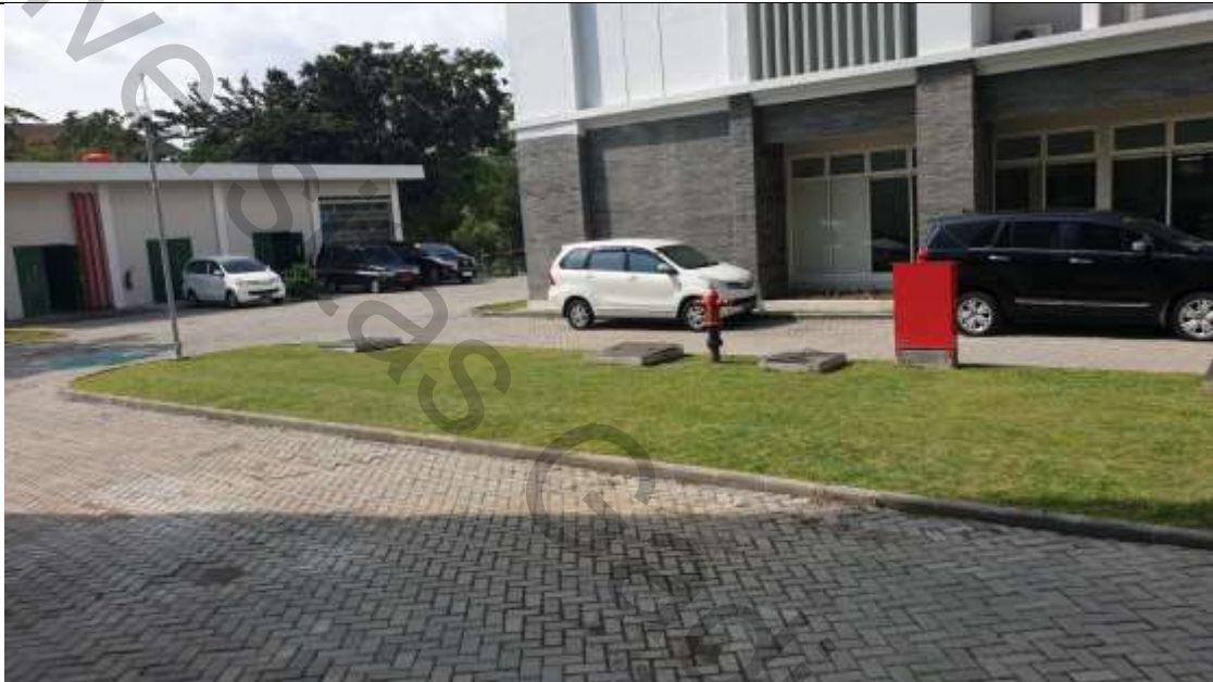
Figure 8 Ground Water Tank in Center for Environmental Study
