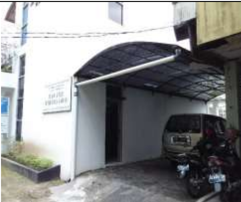
15(n) Injected Rain Water Harvesting in Laboratory of Environmental Engineering
