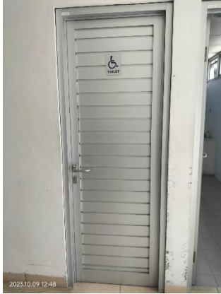
Figure 25 Toilet for Disabled People (People with Special Needs) at Faculty of Geography
