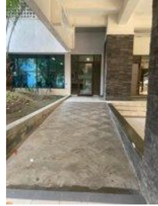
Figure 6 Ramp at Faculty of Agrotechnology
