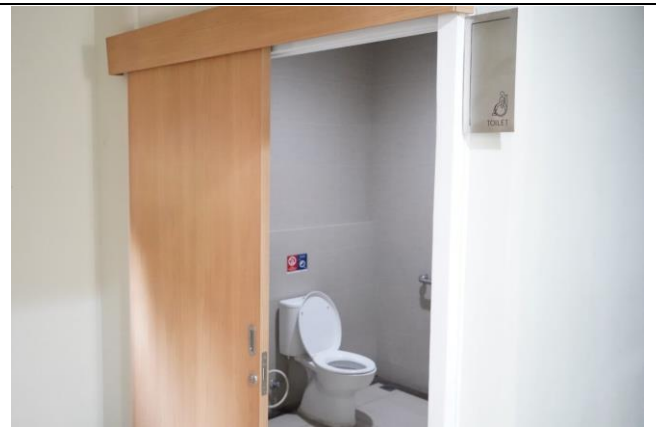
Figure 22 Toilet for Disabled People (People with Special Needs) at Faculty of Agricultural
